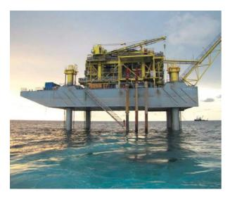
Following refurbishment by Hoondert in the Netherlands, the topsides headed for West Africa on the hull of another of Overdicks innovative self-installing leg barges. The Sanaga 01 module, with its elevated hull supporting an 1800t wellhead platform, was eventually installed in 17m of water offshore Cameroon in April this year.
